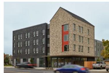
ABOVE NHA's Buri BLDG is located in Portland's growing Gateway District, close to the Gateway Transit Center, and is primarily made up of studios and 1-bedroom units.
